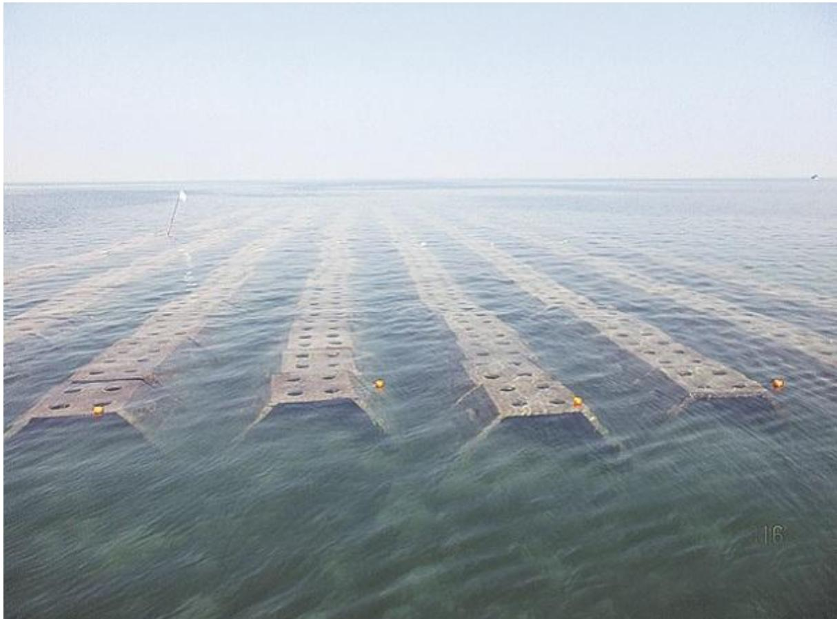
The plan was to deploy artificial reefs near Vaan in such a manner that they would reduce the impact of high-energy waves hitting the island. There was also hope that the artificial reefs — trapezoidal perforated structures fashioned out of ferro-cement and steel — would become home to new coral colonies and fish production.
